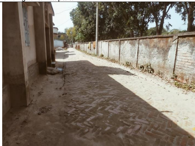
R-8 Improvement of Road from Monowar Mia House to Shishirpara BC Road near Khalek rice mill Back side of Upazila Parishad at Mohila College para, Ward no 02 & 08.
