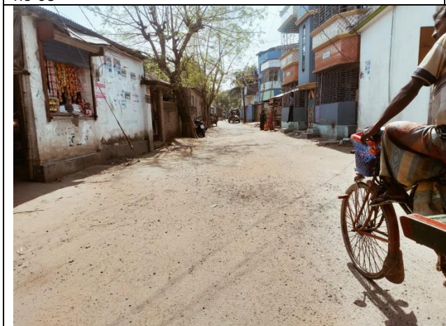
Road-10, Improvement of Road from kushtia-meherpur RHD near post office to chowgasa boro mosque near kathuli BC road Ward no 04
