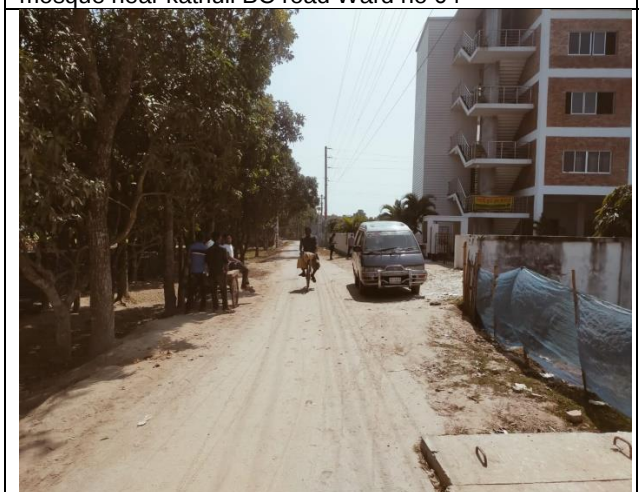
Road-11, Improvement of Road from sandhani school and college to maidir canal, including Cross Drain
