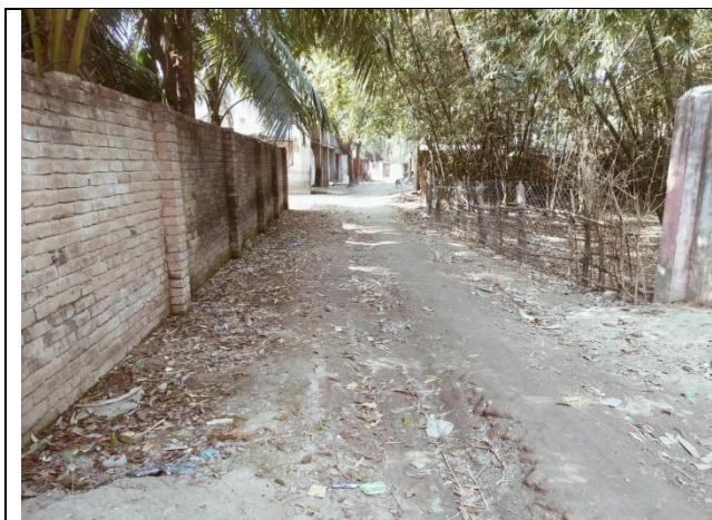
R6.Improvement of Road from R&H road to Fataipur Graveyard
