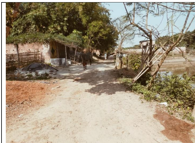
Road-9, Improvement of Road from Nazir Baniyas house to maidir math at paschimpara malsadoh, Ward no 05
